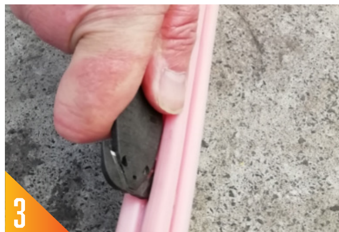
Web Slitting Tool used to separate drop microduct from bundle.
