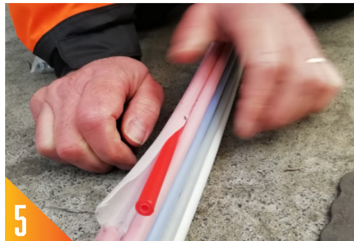
Sheath easily removed by hand.
