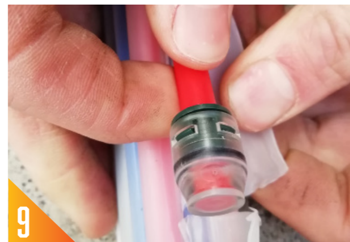
"Dead end" of the microduct is end capped.
