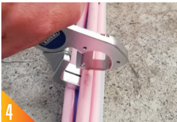
Conduit is cut at a distance ahead to allow for enough length to perform the drop using appropriate tool.
