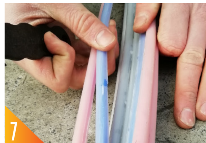
Multiple drops can be separated from the bundle in one go.
